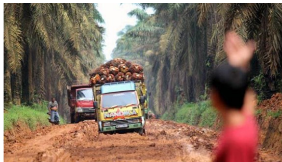
Figure 4. Condition of unpaved peatland infrastructure during the monsoon season
